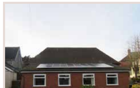
Solar panels installed
